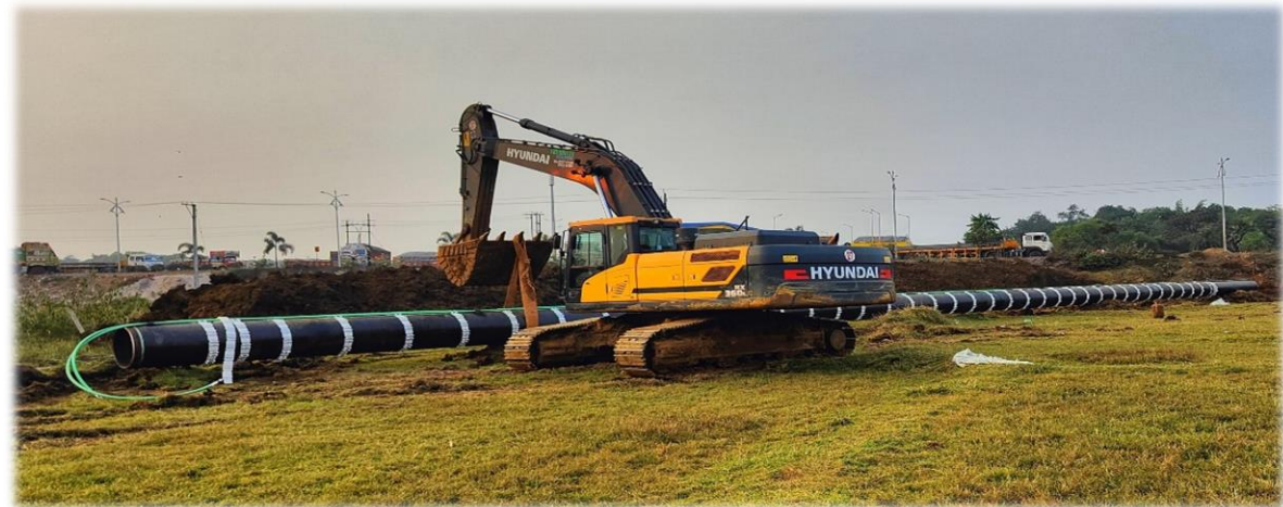
Setting up slurry pipeline
