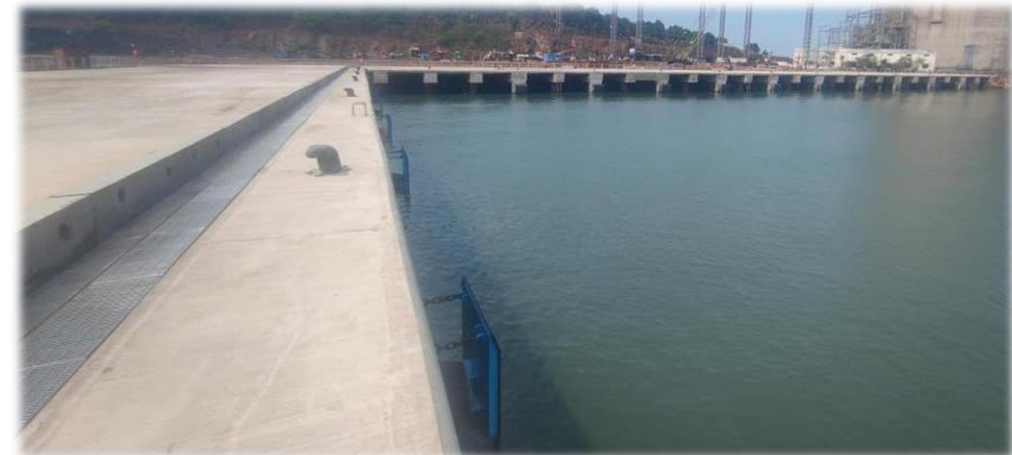
Expansion work at Jaigarh Port
