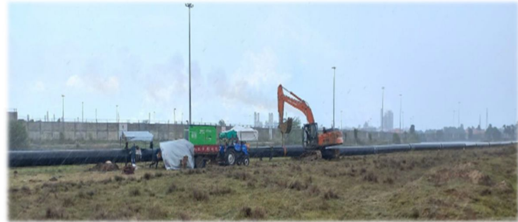
Setting up slurry pipeline
