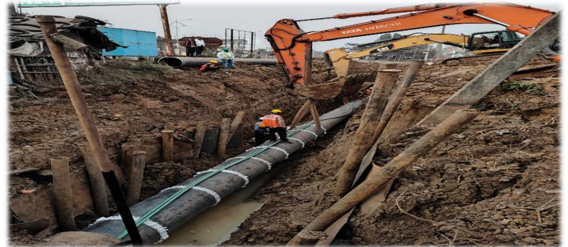
Setting up slurry pipeline
